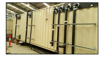
Minimal site-fabricated piping
