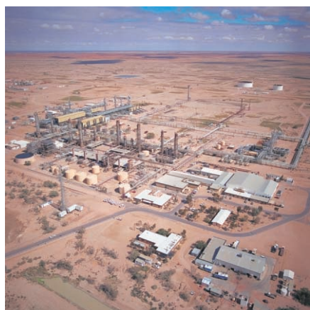
Moomba gas and liquids processing plant, Cooper Basin. (Photo 43803)
